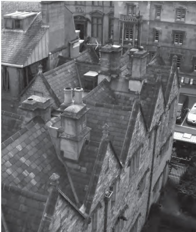
The Kettell Hall roof from scaffolding on Staircase 5
